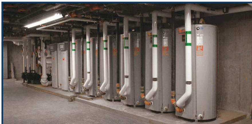
Domestic and pool hot water exchangers and heaters.
